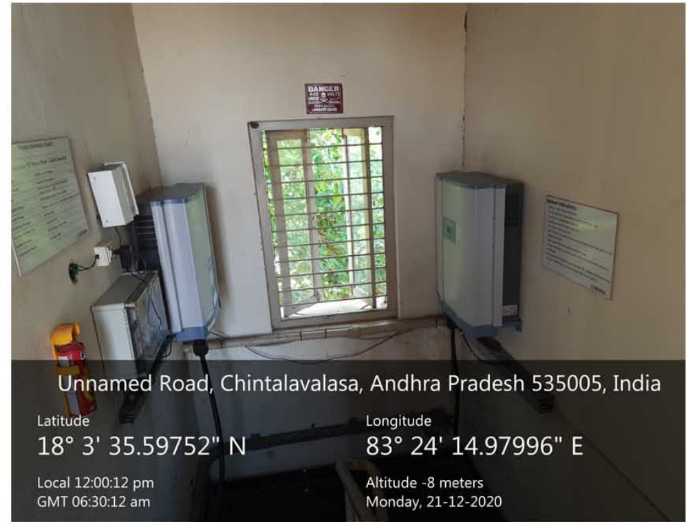
75Kwp Plant located on rooftop of ECE department and associated Inverters
