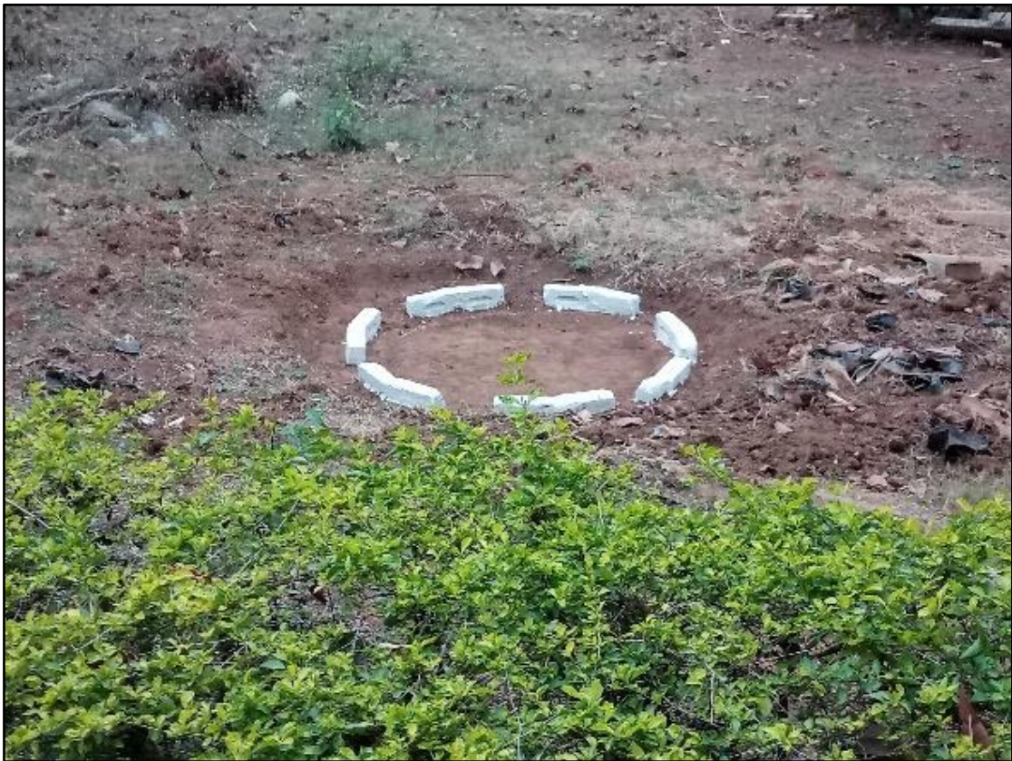
Rain water harvesting pits
