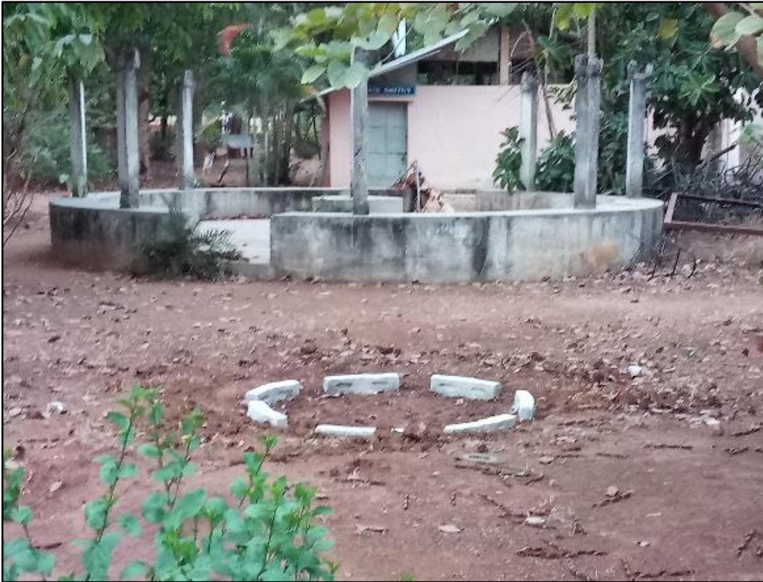
Rain water harvesting pits
